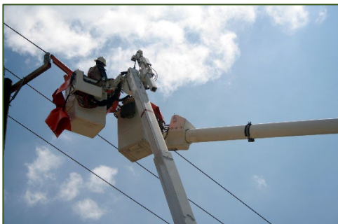
Shown: Utility Workers Using Bucket Trucks
