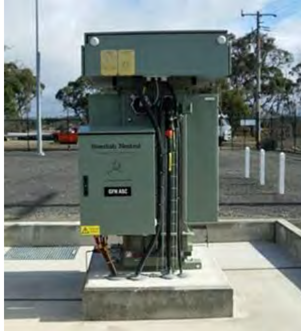
FIGURE PG&E-7.3.3-5: ARC SUPPRESSION COIL / GFN
