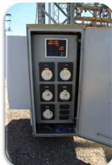
Analog Relay Equipment
