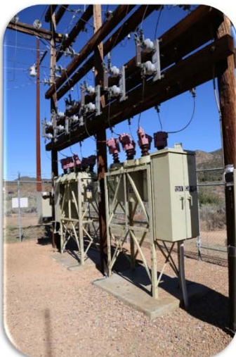
Oil Circuit Breakers
