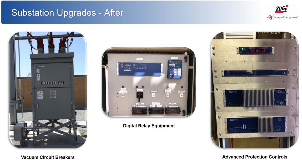
Figure 4 Newly Installed Substation Advanced Protection Equipment which supports the FCP Pilot
