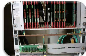
Aging Remote Terminal Units
