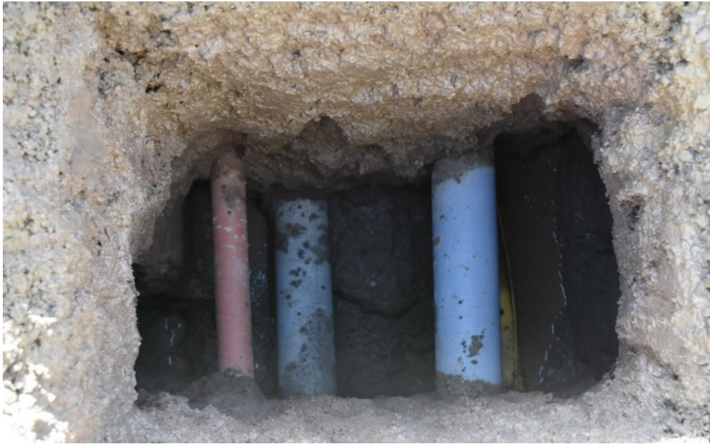
Figure 11: Potholes, such as this one, provide windows to determine the exact location of pipelines prior to excavation across the entirety of a project.
