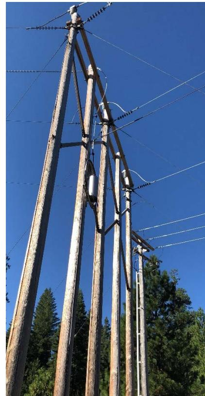
*60kV wood pole design with 4kV riser pole for undergrounded segment of the line*
