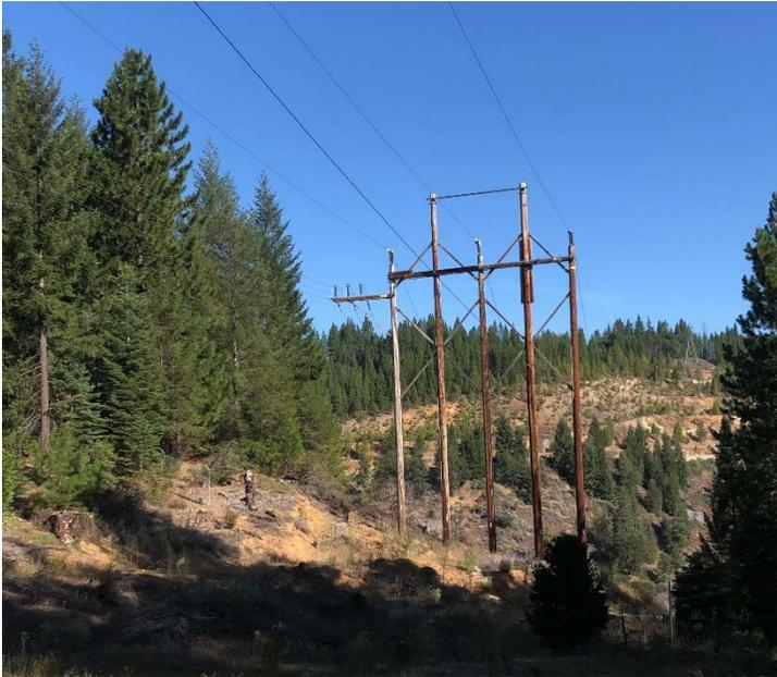
*60kV wood pole design with 4kV attachment*
