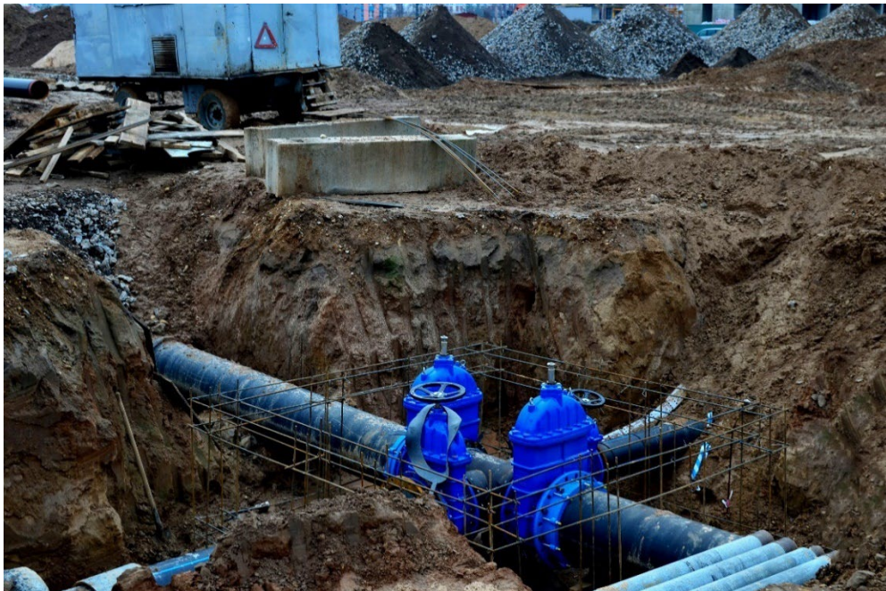
Figure 7: A pipeline with valves is installed in the ground.
