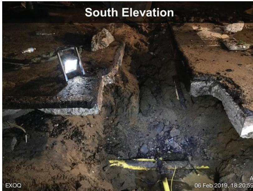
**Figure 7:** (from **Exh 13**) Damage at branch connection. Courtesy PG&E.
