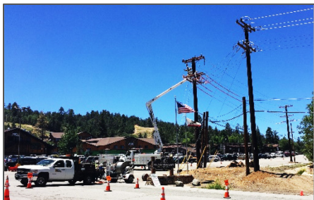
Pole replacement in Bear Valley Electric Service, Inc.
