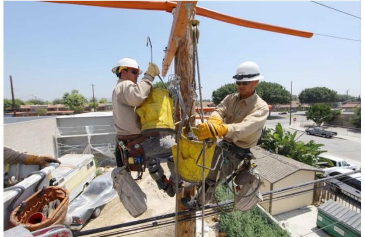
Pole-loading Inspection (Image courtesy of SCE)
