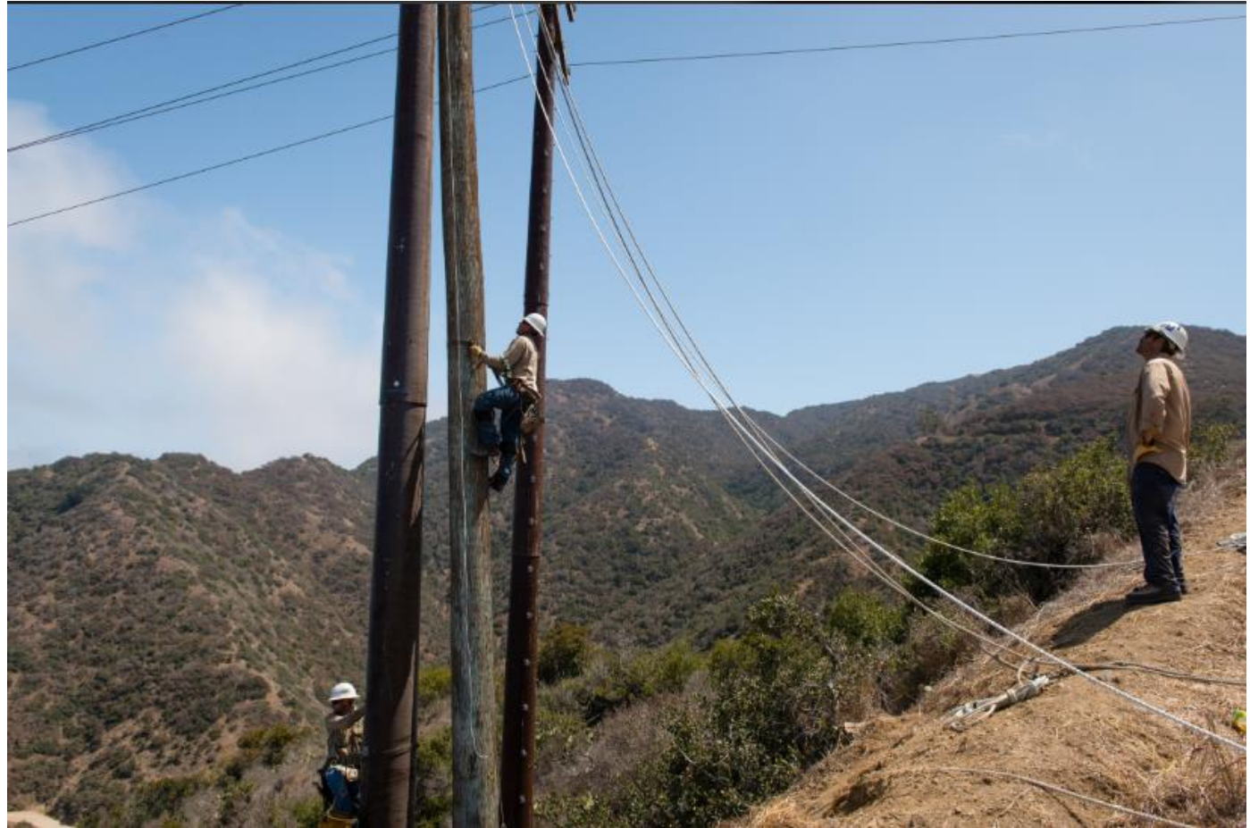
Fiberglass composite pole installation
