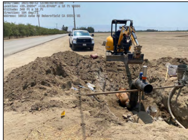
Repair of leaking concrete pipe outside of Bakersfield. Image provided by pipeline operator. From Investigation 21LA01474.
