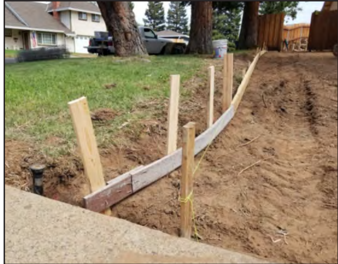
Closeup of new driveway excavation performed by C-8 Concrete specialty contractor. From Investigation 21SA01473
